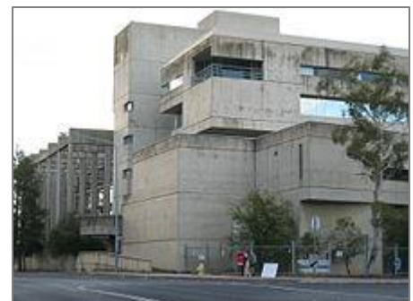
Figure 5 : The Cameron Offices
