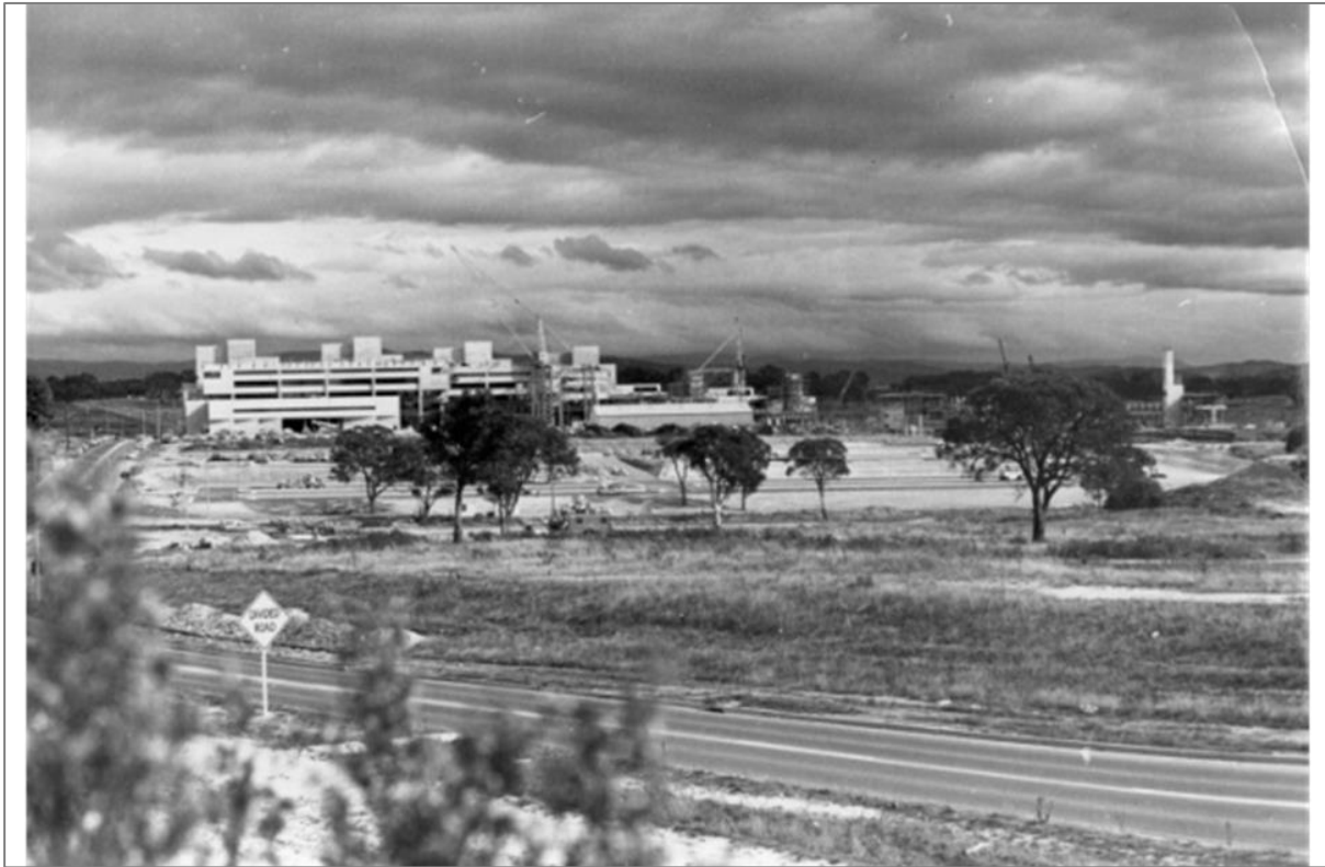
Figure 56: Progress on the Construction Site dated 15 May 1974
