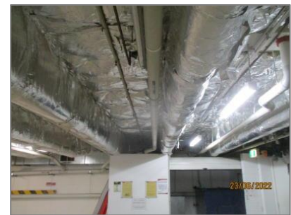
Figure 35 : Foil wrapped structural beams
