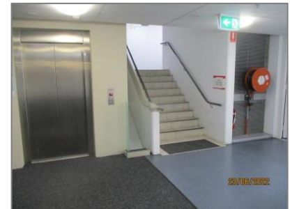
Figure 29 : Lift and Stairs
