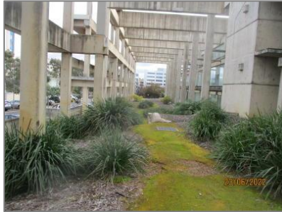
Figure 40 : View along courtyard Wing 5
