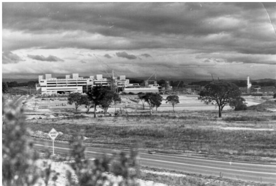
Figure 11: 15 May 1974 Progress on the Construction Site 35
