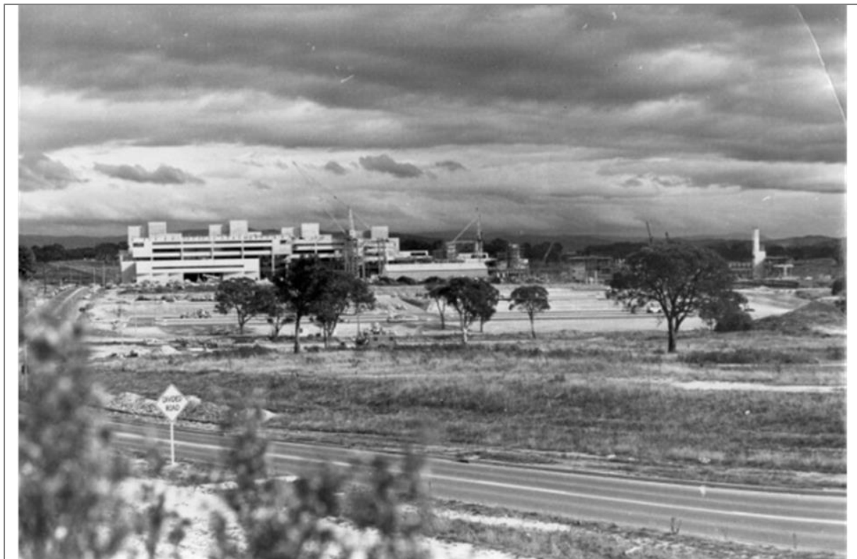
Figure 30: Progress on the Construction Site dated 15 May 1974
