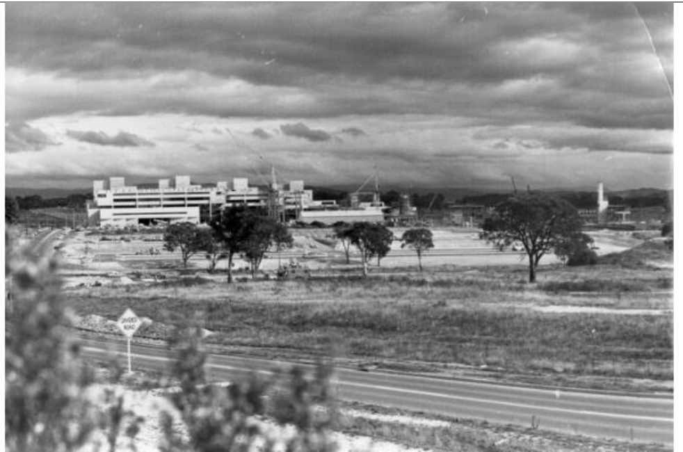
Figure 16: 15 May 1974 Progress on the Construction Site
